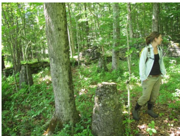
Photo 55: Cement pillars at the edge of the Swamp. Most likely, they were erected to raise the wooden floor of a hay barn above the periodically wet ground.
